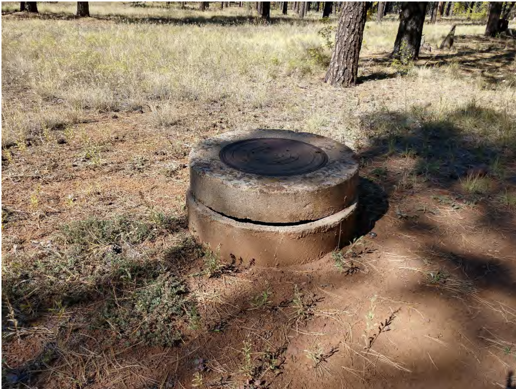
Photo 10 Man-hole access to City of Flagstaff water line.
