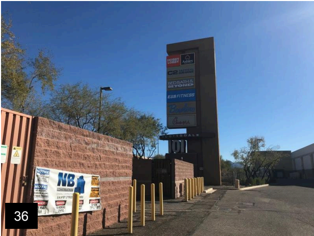
36 Second cell tower and battery storage enclosures
