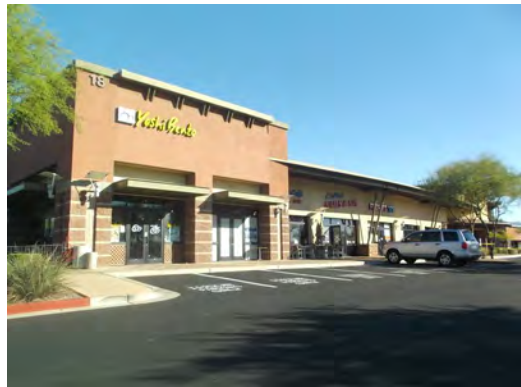
PHOTO #10 SOUTH ELEVATION, F BUILDING
