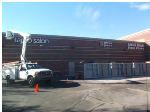
PHOTO #6 NORTH ELEVATION, B BUILDING
