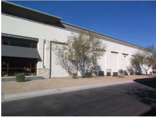
PHOTO #7 EAST ELEVATION, B BUILDING
