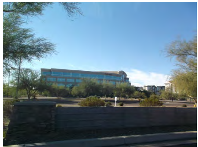
Adjacent property south - East Mayo Boulevard, followed by office building
