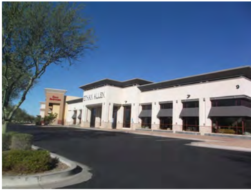
PHOTO #1 SOUTH ELEVATION, ETHAN ALLEN
