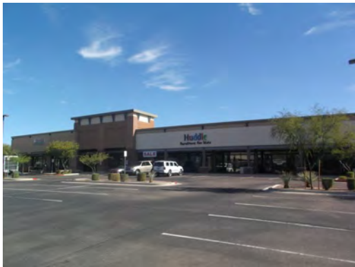
PHOTO #9 WEST ELEVATION, C BUILDING
