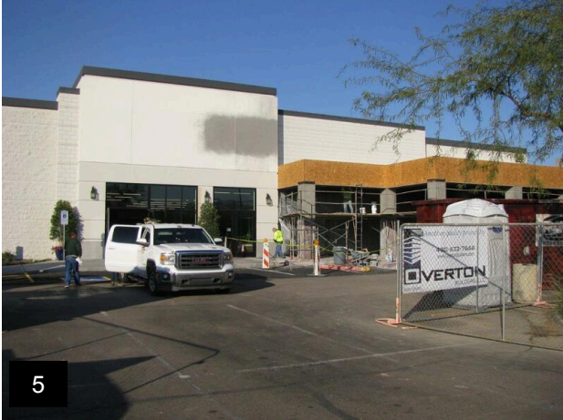
5 Building undergoing tenant improvements
