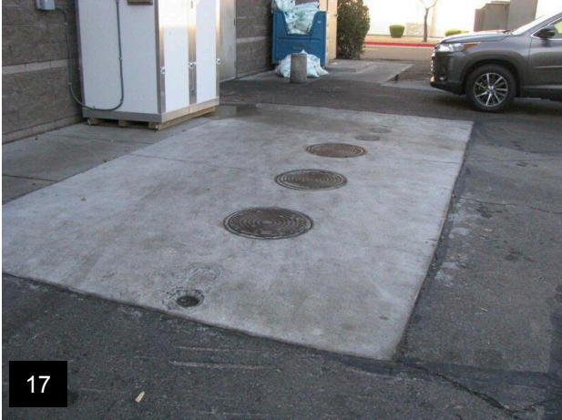
17 Typical grease trap
