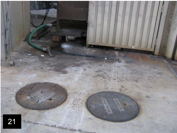
Hose draining compactor behind Harkins theaters
