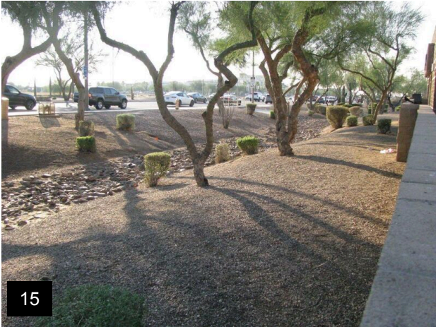
15 Stormwater retention area
