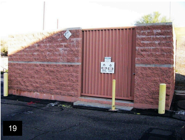
Verizon diesel generator enclosure
