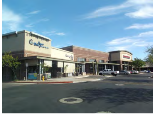
PHOTO #8 SOUTH ELEVATION, B BUILDING
