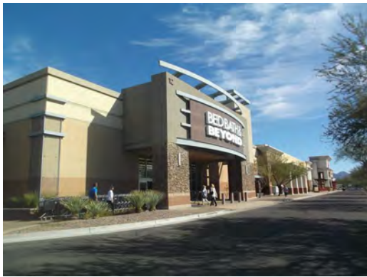
PHOTO #3 SOUTH ELEVATION, BED BATH & BEYOND
