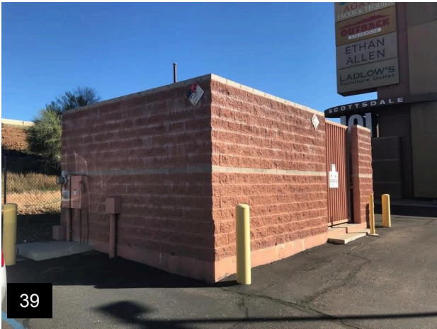
Vent pipe for emergency generator
