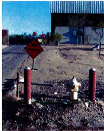
Hydrant south of Transfer Building
