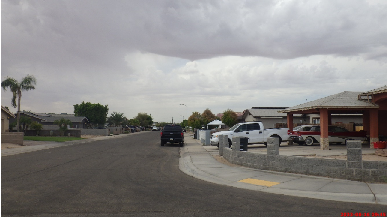
View from the southern project limits looking south along Ed Pastor Avenue.
