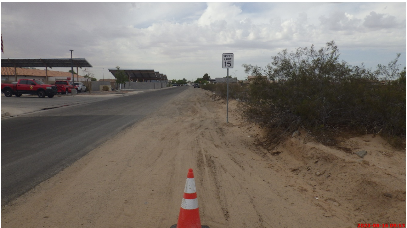
View from the eastern project limits looking south along McCain Avenue.
