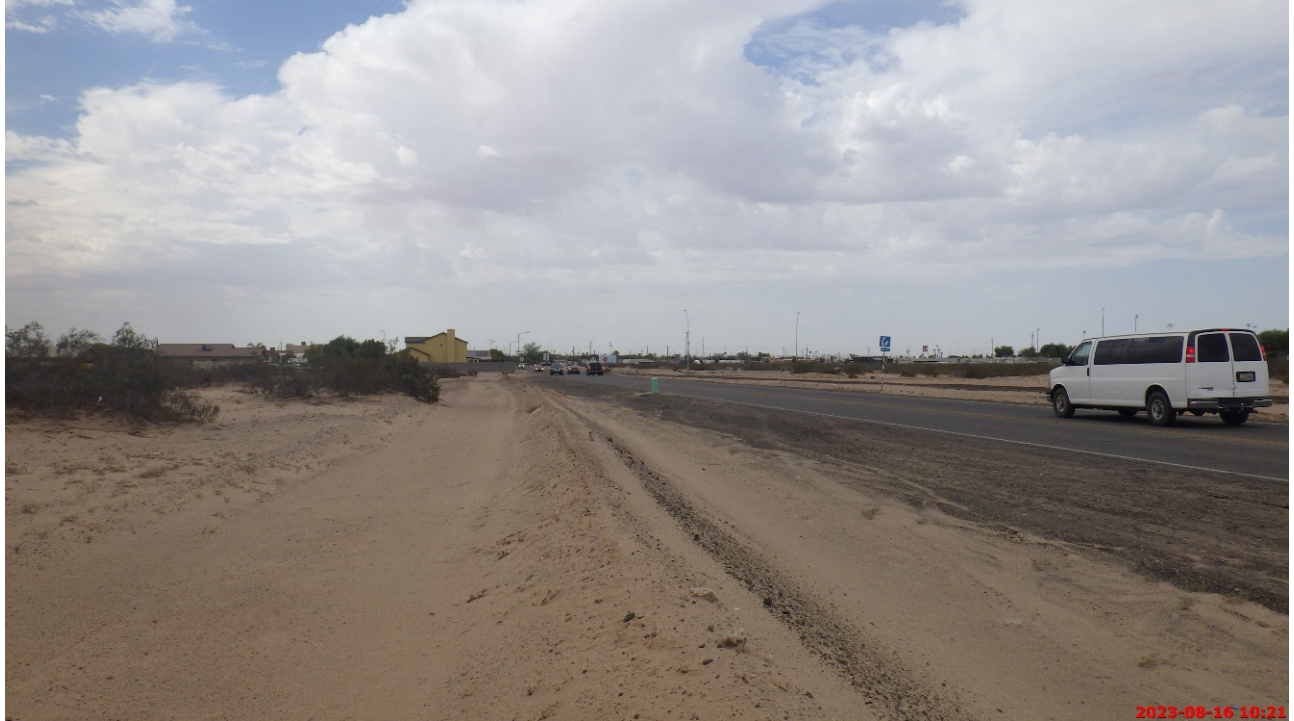
View from the western project limits looking south along 4 th Avenue.
