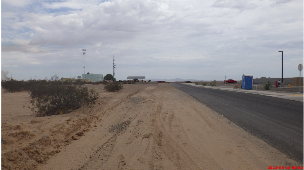
View from the eastern project limits looking north along McCain Avenue.
