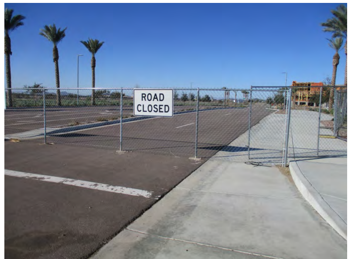
Photograph 20 – A view of the new 4-lane paved drive, looking west-southwest.
