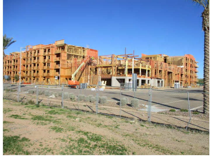
Photograph 18 – A view of the north adjoining building under construction, looking northwest.
