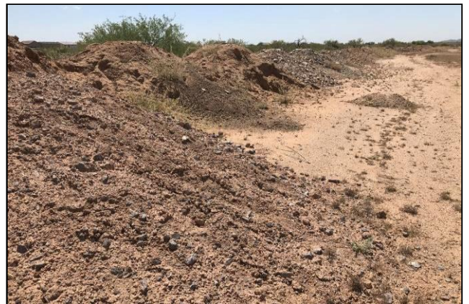
Picture 12 - The piles of soil, gravel, and concrete rubble that followed the west Property boundary.
