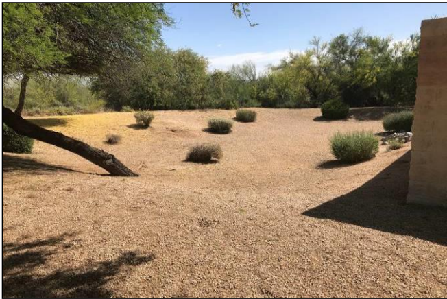
Picture 9 - One of the two retention basins observed near the lift enclosure. No staining was noted.
