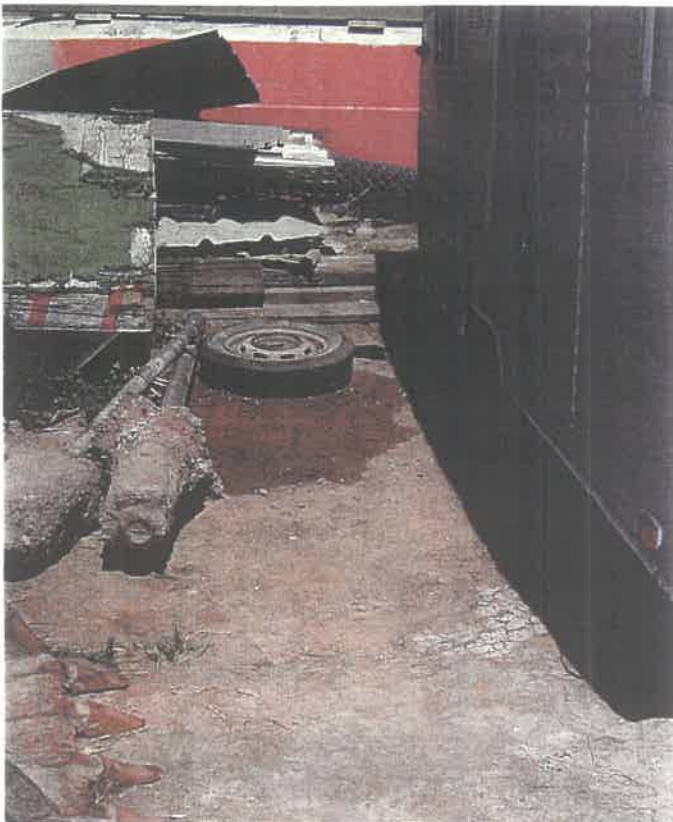
Oil Tank Stains
