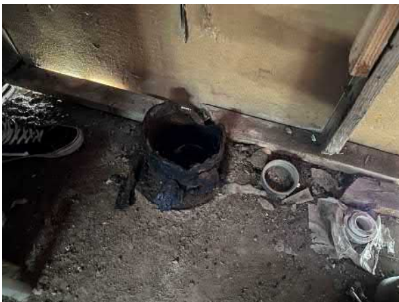
Photo #35 View of a groundwater well located in the central storage area.
