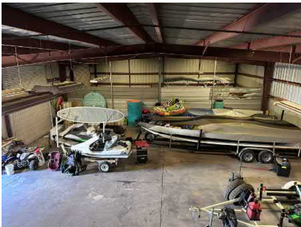
Photo #11 View of the interior of the western storage building.
