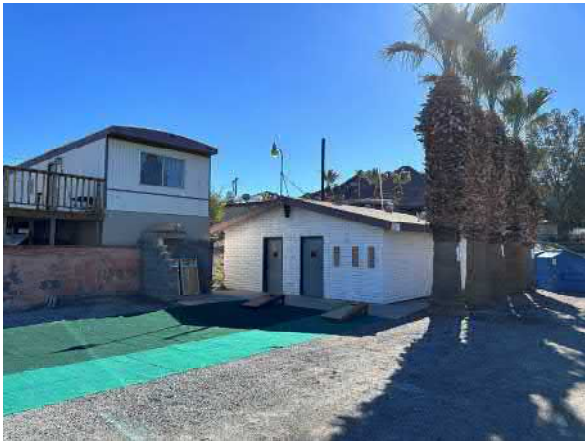
Photo #9 View of the restroom and shower building.
