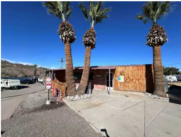
Photo #5 View of the Shipwrecked Pirate Bar and Grill located on the central portion of the site.
