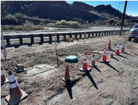
Photo #27 View of the southern septic holding tanks.
