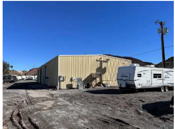
Photo #10 View of the storage building located on the eastern portion of the site, looking north.
