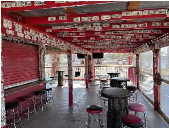
Photo #9 View of the southern bar building located on the western portion of the site.
