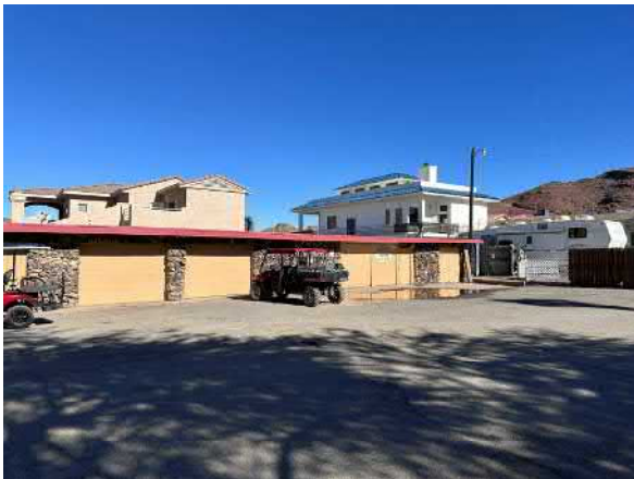
Photo #5 View of the storage and maintenance shop located on the northern portion of the site.
