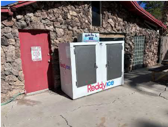
Photo #7 View of the kitchen and restaurant building located on the western portion of the site.
