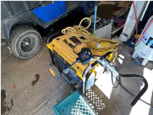
Photo #13 View of the portable 900-Watt generator located inside the maintenance shop.
