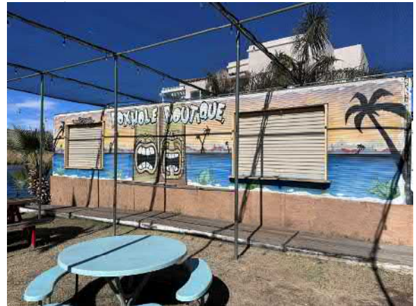
Photo #10 View of the T-shirt Shop Building located on the northwestern corner of the site.
