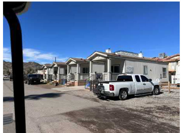
Photo #12 View of multiple rentable modules located throughout the site.
