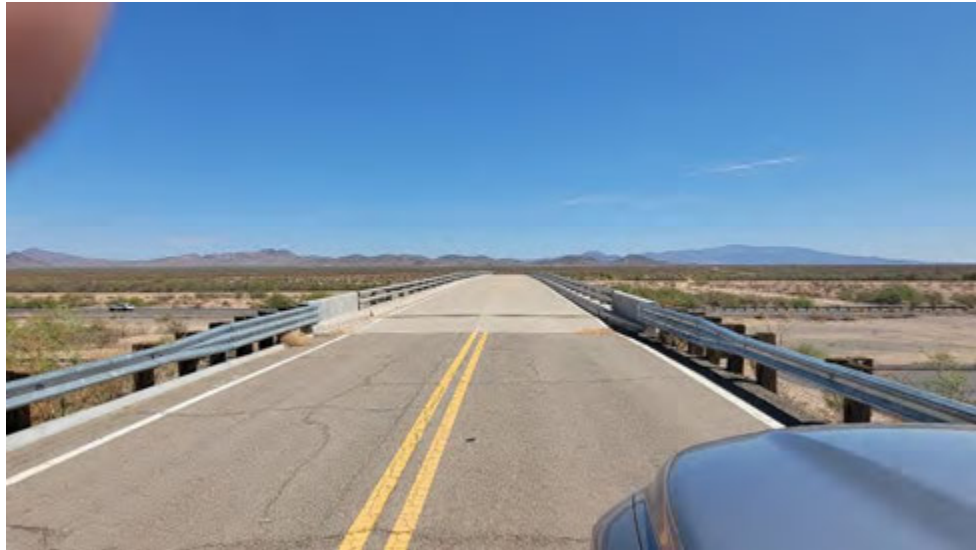
Photo 47: 7-9-22: Sore Finger Road overpass, looking north.
