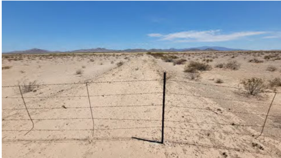
Photo 53: 7-9-22: Looking north from I-10 of the typical levees found on the northwest segment of the Subject Property.
