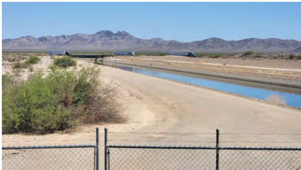
Photo 36: 7-9-22: Looking northwest at the Hayden-Rhodes Aqueduct south of I-10. I-10 in the background.
