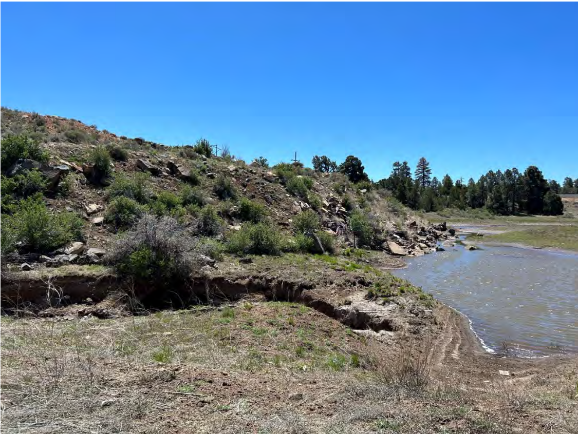
Photo 18 View of debris pushed into Rio de Flag channel from cleared area (up the hill to the left).
