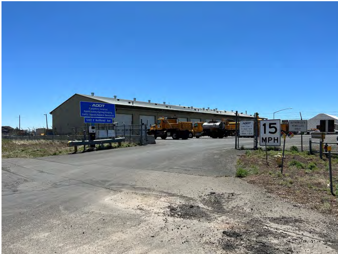
Photo 23 View from Railhead Avenue into ADOT yard north entrance.
