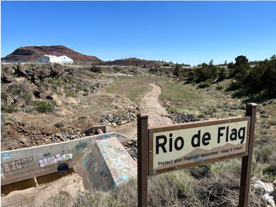
Photo 11 North view of Rio de Flag east of the ADOT yard south entrance.
