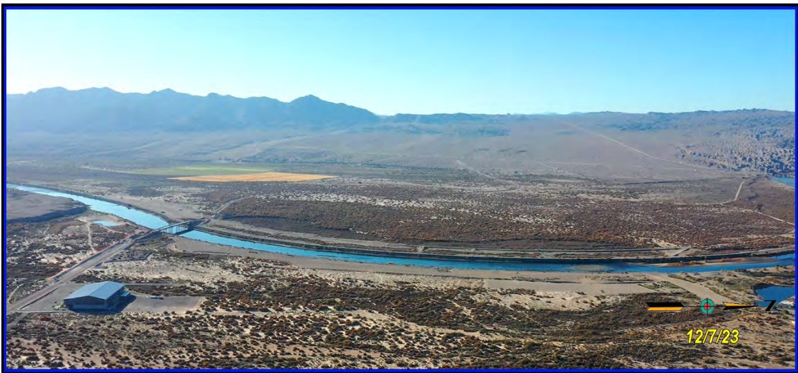
Figure 8 - Aerial Photograph Looking West of the Subject Property
