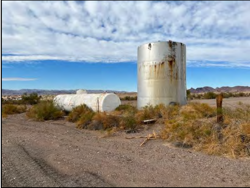
Photo 5: Aboveground storage tanks within the Mohave County Maintenance Yard.
