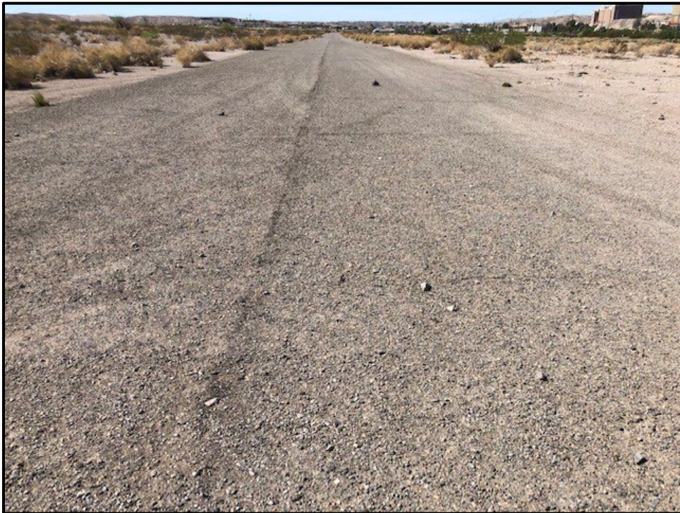
Photograph 2. Remnant of paved runway within the subject property.
