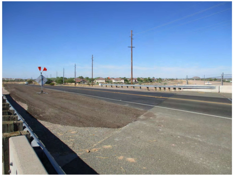
Photo 16 - View of single-family residences northwest of the aqueduct, looking northwest across Southern Avenue from its bridge.
