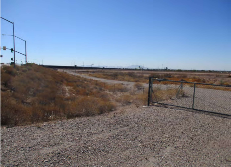
Photo 23 - View of the Superstition Freeway interchange, an aqueduct maintenance access road and the retention basin south of the subject property, looking southeast.
