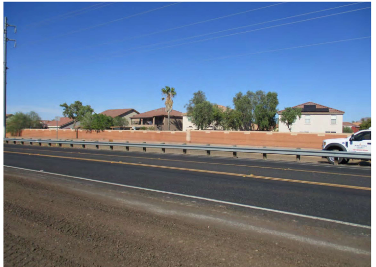
Photo 18 - View of the north adjoining Silverwood single-family residences, looking northwest across Southern Avenue.
