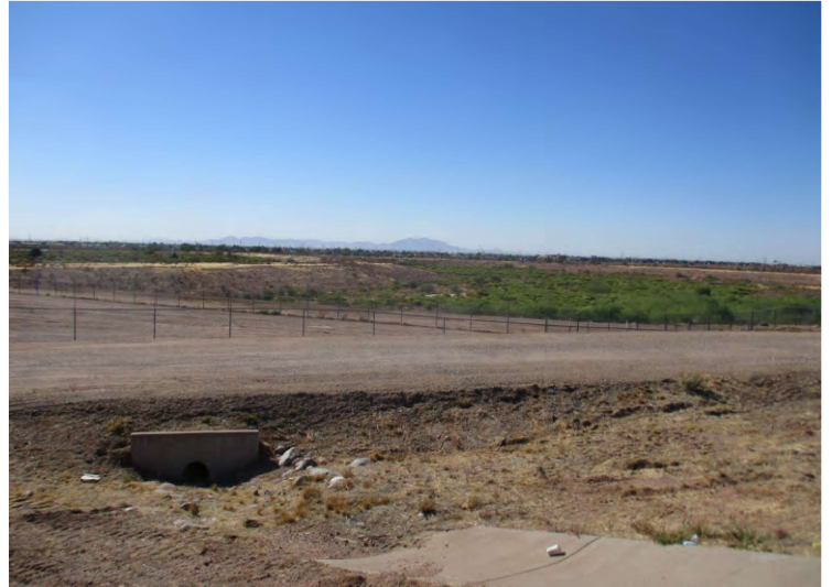
Photo 28 - View of the broad retention basin on the east side of the aqueduct, looking southwest from Southern Avenue.
