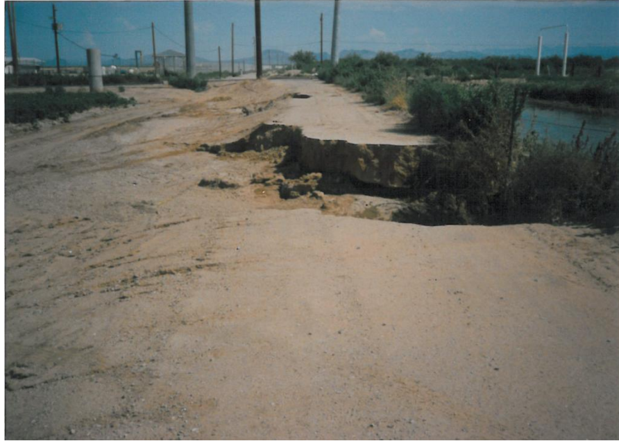
Photo 4: Breach in farm embankment south of Germann Road. Breach occurred during storm event of early 1990s. (Looking north along Meridian Road alignment from south of Germann Road.)
